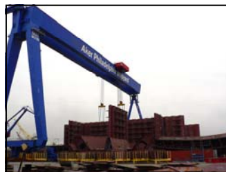
Hull 009 and 010 sections staged north of the Building Dock
