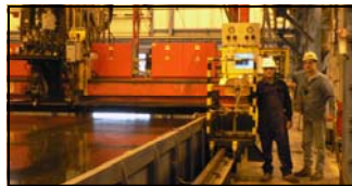
Steel Cutting for Hull 013.
