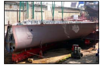
1E11 of Hull 009 is set in the dock.
